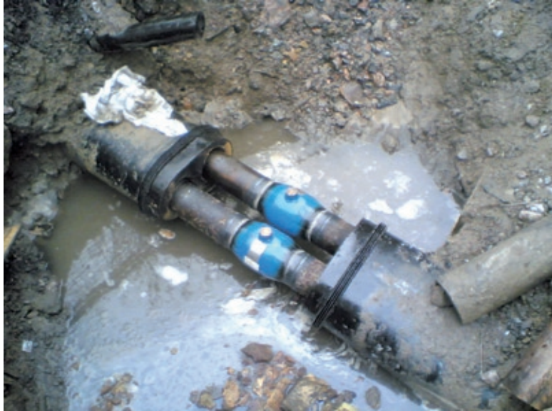
Figure 5: Heating pipe under reparation photographed by Toni
