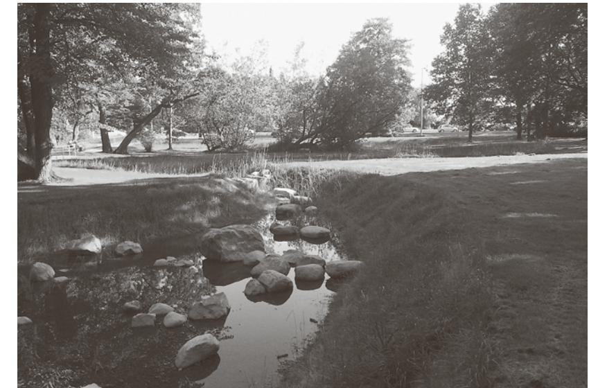
Fig. 12 The Vauhtitie wetland, a new type of GI structure collecting and managing stormwater from a new urban district of Pasila. Located in a park, it enhances the local biodiversity and recreational value.
