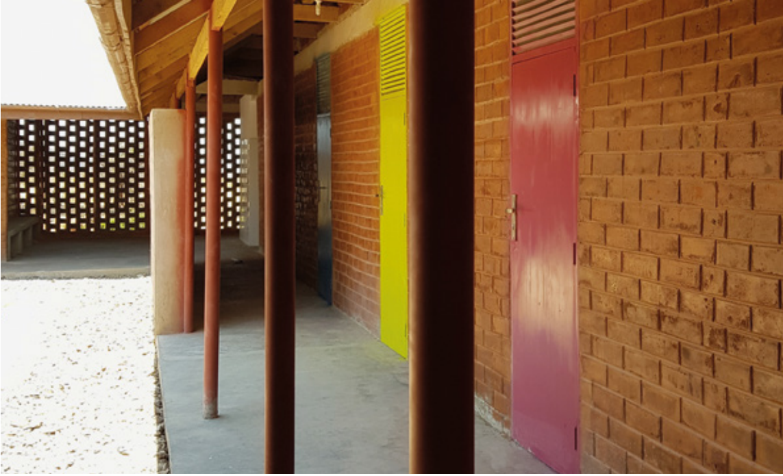
Ventilation wall near the toilet areas in Nyang'oro hostel. PHOTO SAIJA HOLLMÉN/HRS
