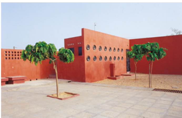
Women's Centre in Senegal: old glass bottles that make glass bricks, rusty car rims as ventilation openings in the toilets, window shutters and doors made of recycled metal. PHOTOS JUHA ILOINEN AND HELENA SANDMAN
