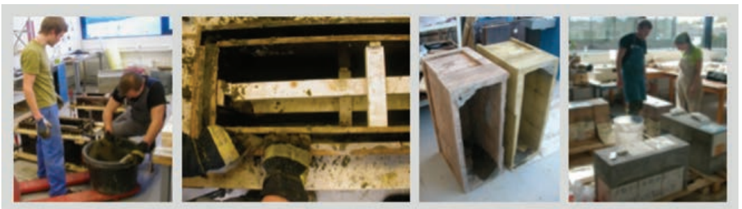
Figure 3. 13: ABCD (left to right) A: Cement mixed with sand and colour. B: The inner and outer construction for making the form of the concrete seating blocks. C: The colored seating blocks with space for tiles. D: Students placing tiles.
