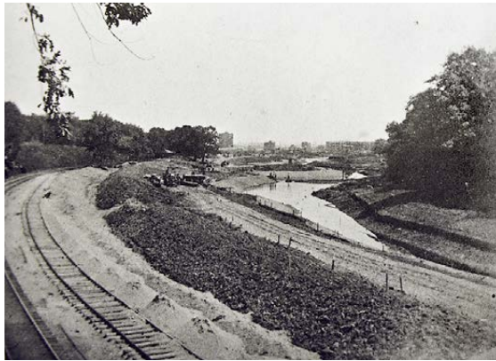
■ Figure 62. Grading in progress in the 1890s on the Muddy River Improvement near Longwood avenue, looking downstream towards Boston. A railway has been constructed to bring the large amounts of landfill to the site. Zaitzevsky 1982 p. 157 fig.122.
