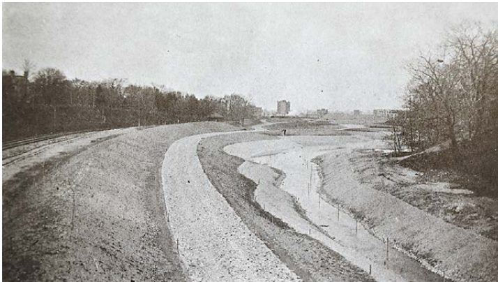
■ Figure 63. Grading nearly complete in 1892, note the sharper meanderings of the river and two stages of leveling. Zaitzevsky 1982, p. 158 fig. 123.
