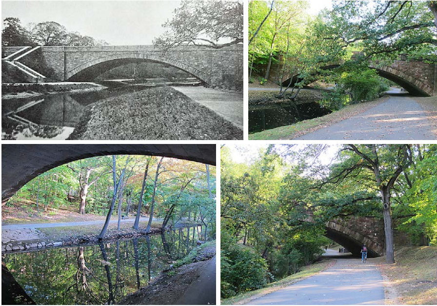
■ Figures 57–60. Muddy River bridges, past and present. Figure 57 shows the Longwood Avenue Bridge in 1901 (Zaitzevsky 1982, fig. 149, p. 175) and in 2014 (Fig. 58–90). The place is very similar today, apart from the vegetation that has grown to make the water's edge on the banks of the river much less depictable. Modern day photos by the author 2014.
