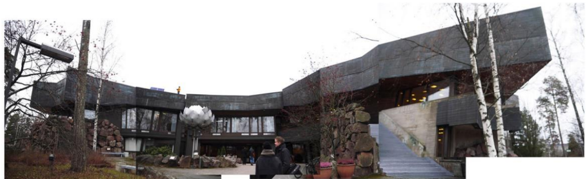
Figure 12. The prototyping experiment view of solar panels placed on the rooftop at 45 degree angles, which left the view "subtly" visible (from Mok and Hyysalo, 2017).
