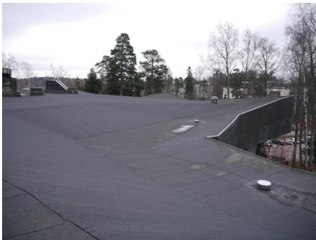
Figure 11. Dipoli's entire rooftop was covered with bitumen felt; photo taken on 13 November 2014 (from Mok and Hyysalo, 2017).
