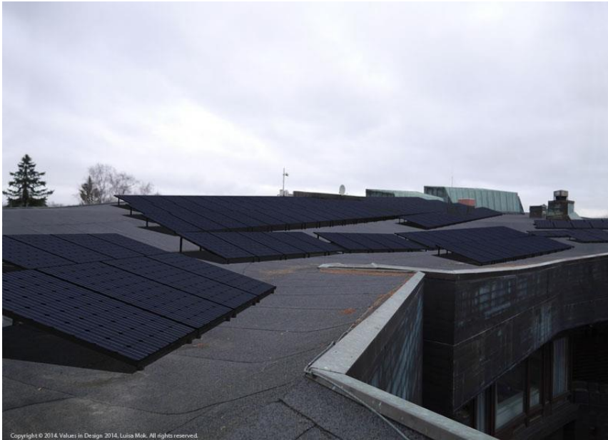
Figure 17. The solar array visible from the rooftop, viewed from another angle (from Mok and Hyysalo, 2017).
