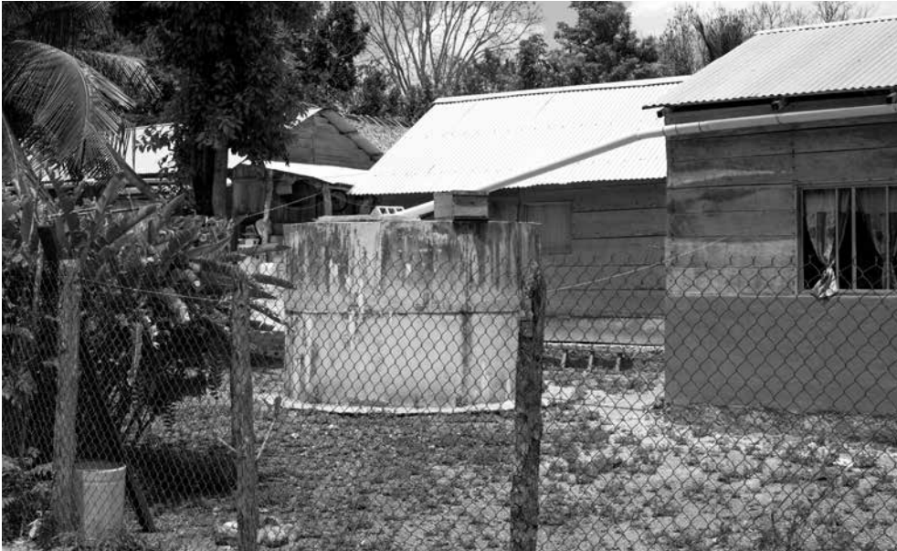
Figure 50. The water harvesting system that most houses in El 20 have, with the 12000 litres water tank, and the PVC tube connected to the rooftop. Photo by Jan Ahlstedt.
