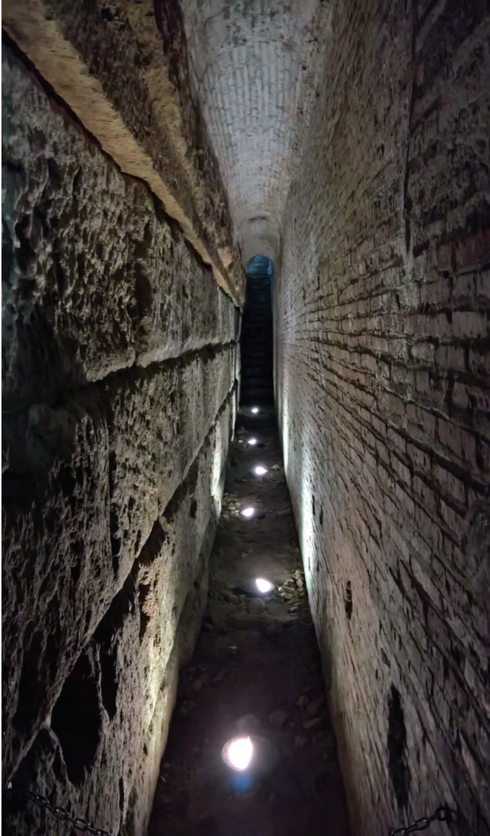
Fig. 1.3.06. The narrow fire alley between the horrea and the domus showing the barrel vaulting resting on the opus quadratum of the horrea .
