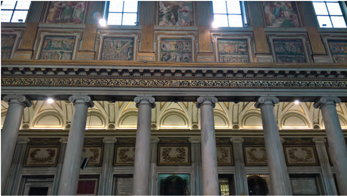
Fig. 2.2.10. Santa Maria Maggiore, detail of the columns and clerestory wall.
