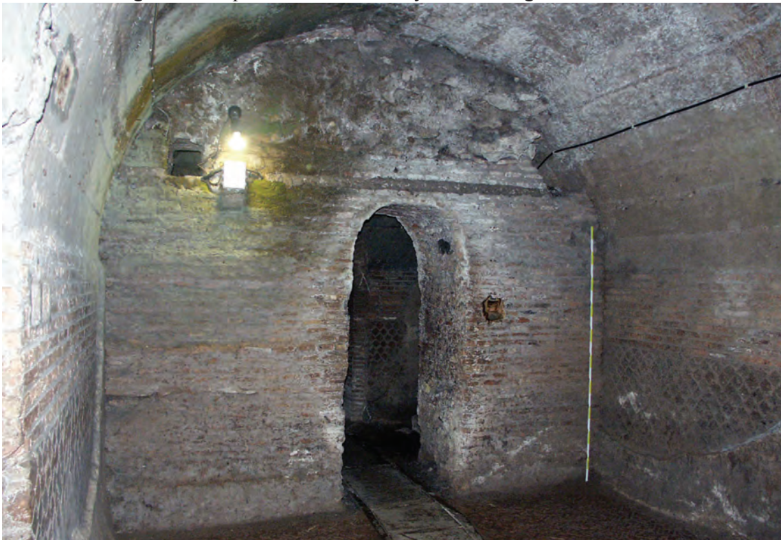
Fig. 1.3.02. Room Y in the horrea showing the load-bearing walls in opus mixtum that carry the vaulting. The narrow doorway is 19th century.
