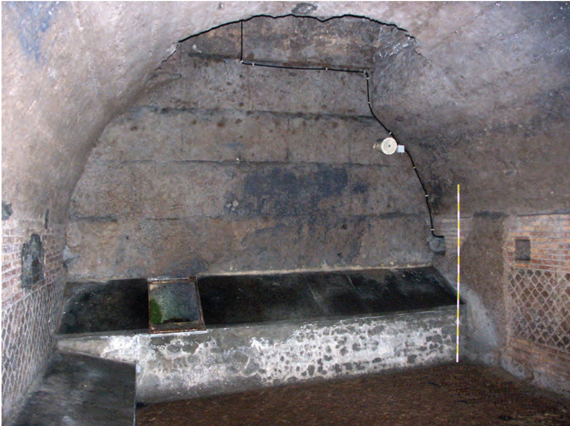
Fig. 1.3.01. Room A1 in the horrea showing the outer envelope of opus quadratum and the load bearing walls in opus mixtum that carry the vaulting.
