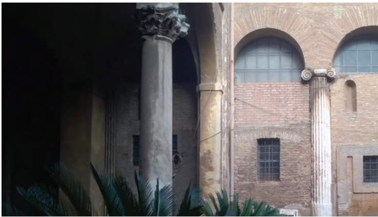
Fig. 2.2.12. Santi Quattro Coronati, the Carolingian northern clerestory wall and columns.
