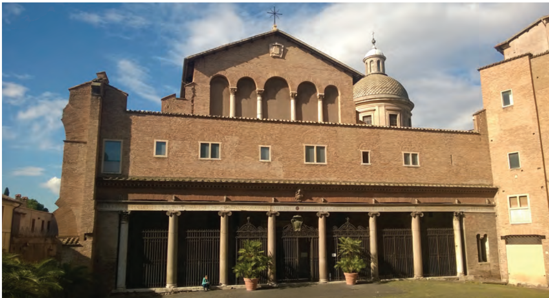
Fig. 2.2.14. Santi Giovanni e Paolo. The narthex is from 1158, but the five arches in the upper part of the nave were restored visible in the 20th century. The five arches repeat the same theme seen in late antique architecture, i.e., making the central arch larger than the rest.
