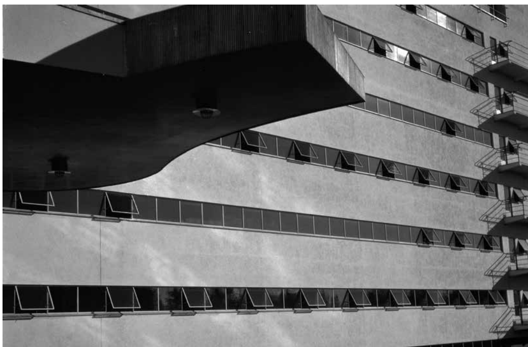
Fig. 1.1g. The canopy covering the main entrance evolved during construction and became asymmetrical. In the background, the ribbon windows of patient corridors. Photographer Aino Marsio-Aalto, 1932. Photo No. 50-003-162. AAM.
