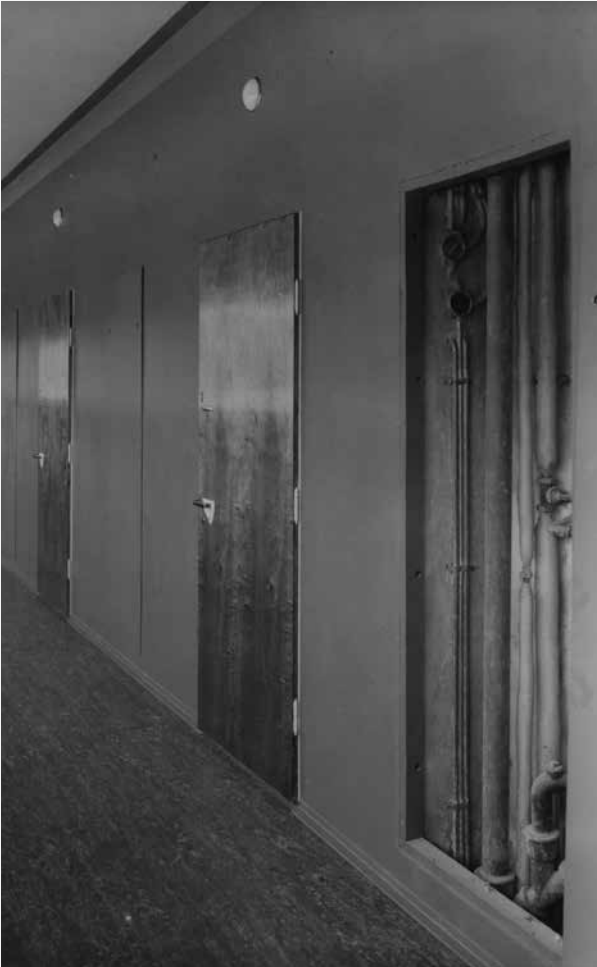
Fig. 3.5.4k. The risers were contained in the wall between the patient room and the corridor, and their service hatches opened into the corridor. Servicing therefore did not require entering the patient room. Photo No. 50-003-153. AAM.
