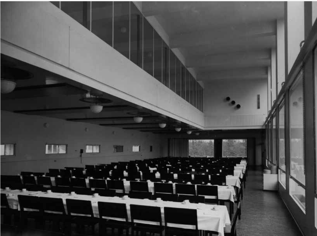
Fig. 3.3.2d. Dining hall. The top part of the back wall housed the film projector. A panel radiator was mounted on the back wall and beneath the glass wall. The encased radiator heaters were mounted on the suspended ceiling. Windows were added to the north-facing wall as demanded by the medical experts. Photo No. 50-003-401. AAM.
