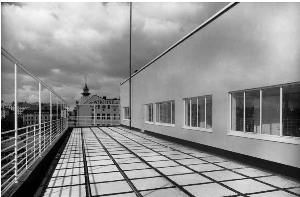
Fig. 2.3b. Turun Sanomat Newspaper Building roof terrace. Photographer Gustaf Welin, around 1929. Photo No. 62-005-083. AAM.
