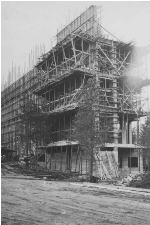
Fig. 3.3.3b. The skeleton of the building was cast in situ floor by floor. Photo PSA.
