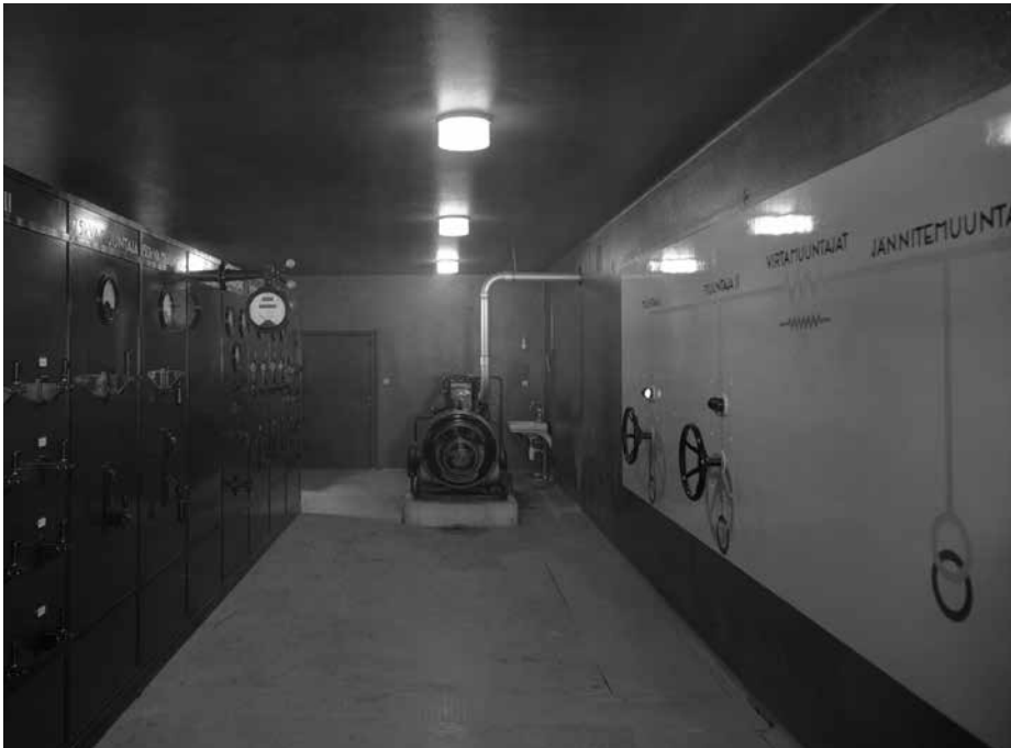
Fig. 3.6.2a. View of the transmission room. Photo No. 50-003-405. AAM.
