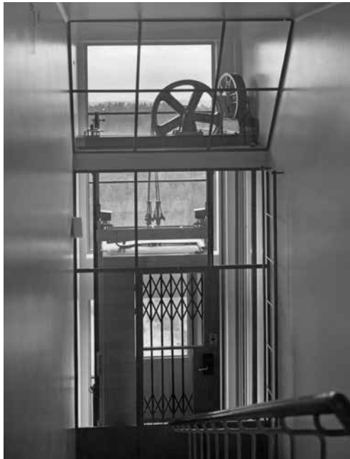
Fig. 3.6.2b. The lift shaft enclosed by glass walls at the other end of A wing. Photo No. 50-003-505. AAM.
