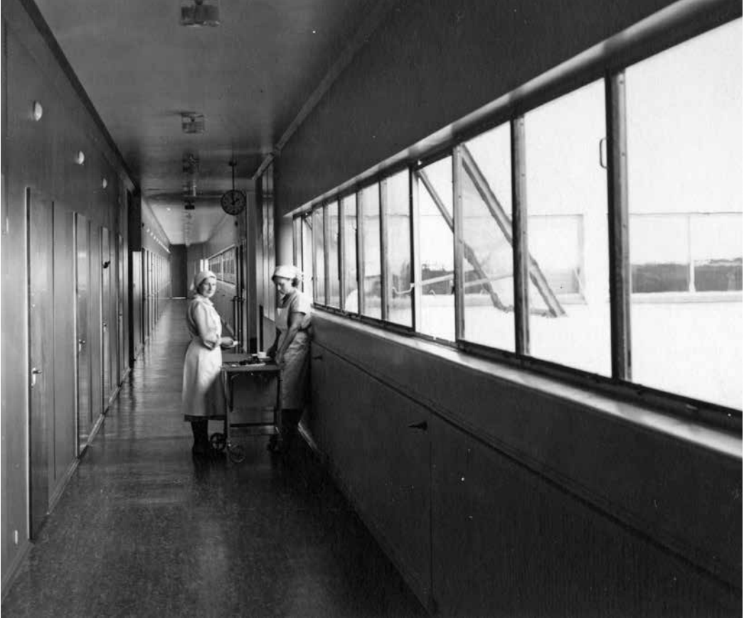
Fig. 3.4.2a. The patient wing corridor is nearly 100 meters long. Photograph No. 50-003-330, photo from the 1930s. AAM.
