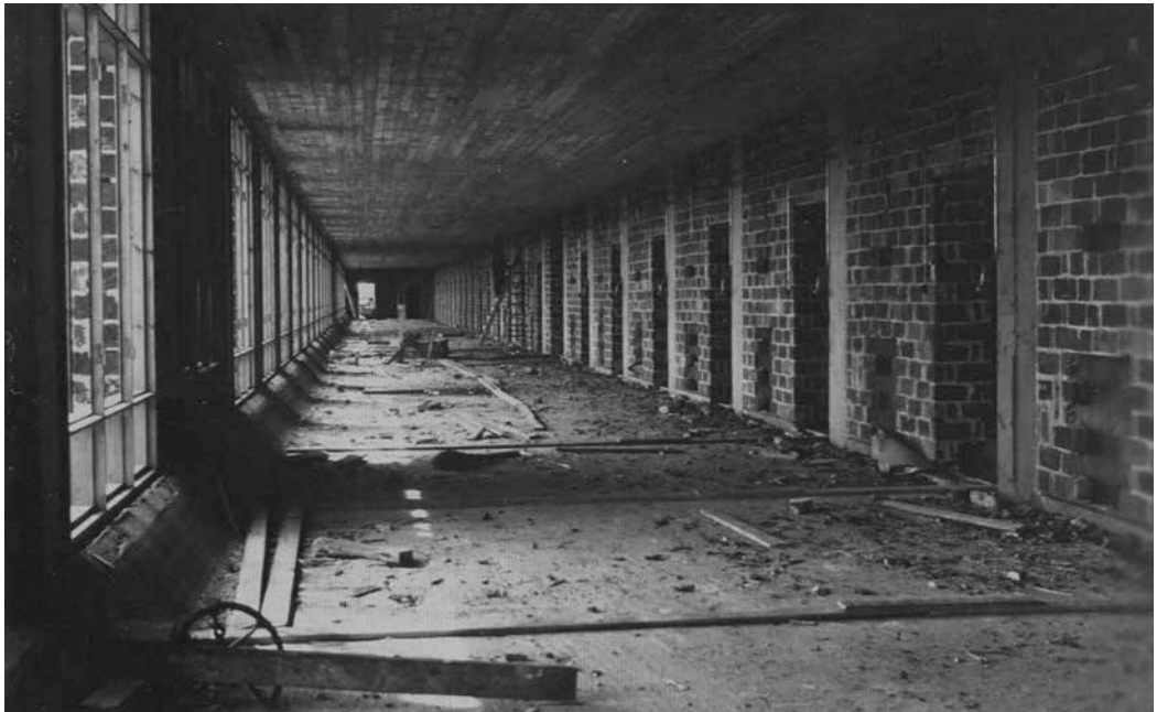
Fig. 3.3.3a. The image shows the floor curving up towards the window in the patients' rooms under construction. The load-bearing pillars in the corridor wall. Photo PSA.
