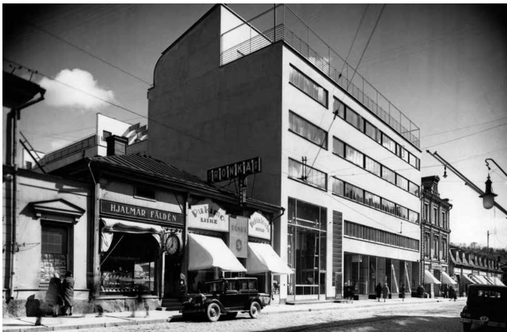
Fig. 2.3a. Aalto applied all the five points of new architecture defined by Le Corbusier to his design of the Turun Sanomat Newspaper Building. Photographer Gustaf Welin, around 1929. Photo No. 62-005-040. AAM.
