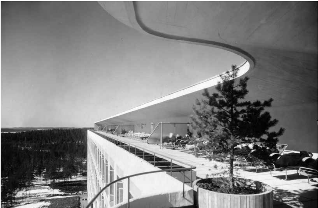
Fig.1.1f. The sundeck. Photographer Gustav Welin, 1933. Photo No. 50-003-265 AAM.
