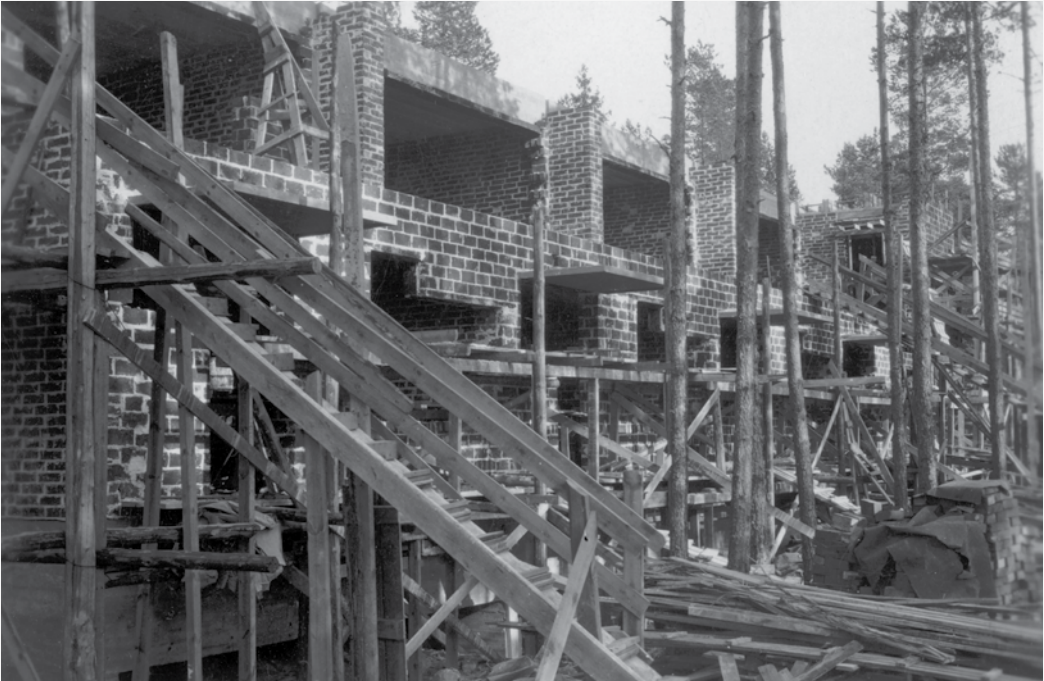
Fig. 2.7a. The photograph of the building site of the workers' apartment building at Paimio Sanatorium appeared in the Rationelle Bauungsweisen (Rational Site Planning) publication and was shot in July 1930. Photo No. 50-003-512. AAM.
