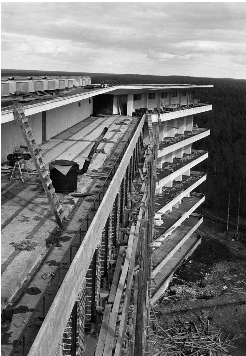
Fig. 3.3.3d. The patient wing building site in autumn 1930. The A wing pillars on the external wall line were cast in situ and protected by a brick layer. Photographer Alvar Aalto or Aino Marsio-Aalto. Photo No. 50-003-079. AAM.
