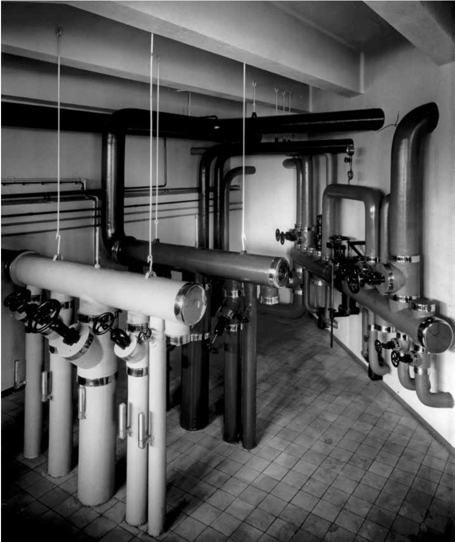
Fig. 3.6.1f. View of the heating system controls. The incoming and outgoing heating pipes at the heating plant were different in colour. Photographer Gustaf Welin, 1933. Photo No. 50-003-411. AAM.
