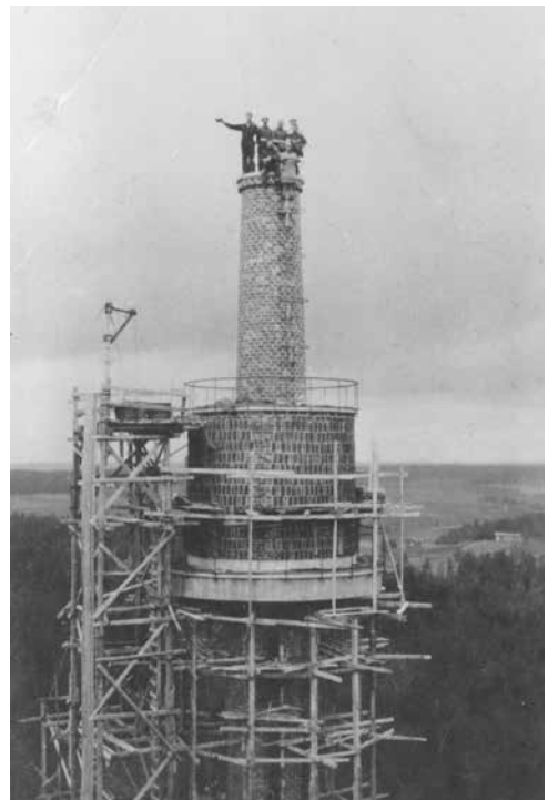
Fig. 3.3.3c. The water storage tank cast from reinforced concrete around the pipe, a delicate work, was constructed only in 1931. Photo PSA.
