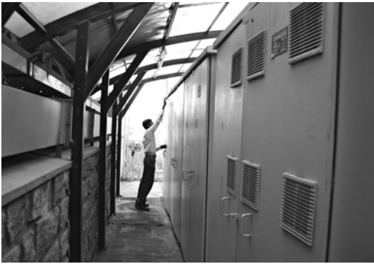
FIG. 04 Madan opening the door of a meter housing in the electric yard.
