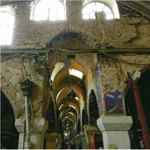
Figures 5.8 and 5.9: Inside the Grand Bazaar, plaster falls off the walls. Instead of once-beautiful murals, the walls reveal bare bricks. Cables bringing power to the shops are attached to the walls haphazardly, with no attention to safety or aesthetics.
