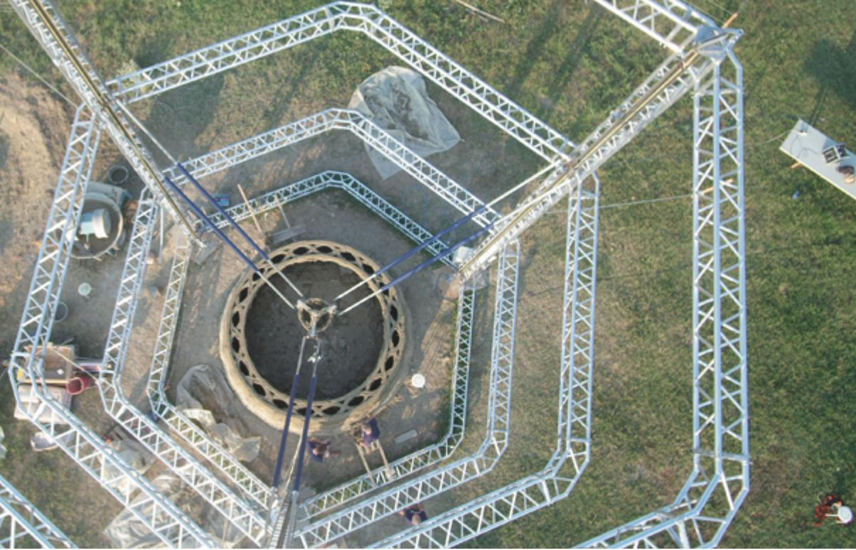
WASProject, Big Delta 3D printer for adobe houses, 3D printer, additive manufacturing, adobe and fluid-dense materials
